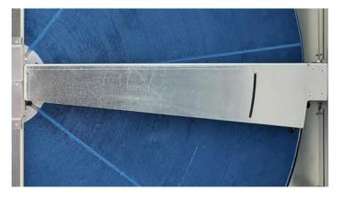
Purge sections minimize cross leakage by shunting a portion of the supply air back into the exhaust air stream and can limit cross leakage to less than 1%. Studies have shown that changing the purge angle from 0° to 12° has only a small impact on the effectiveness (energy transfer) of the energy conservation wheel (2%-3%), while the reduction in gaseous carryover is substantial. The degree to which the purge angle should be adjusted is dependent on:
